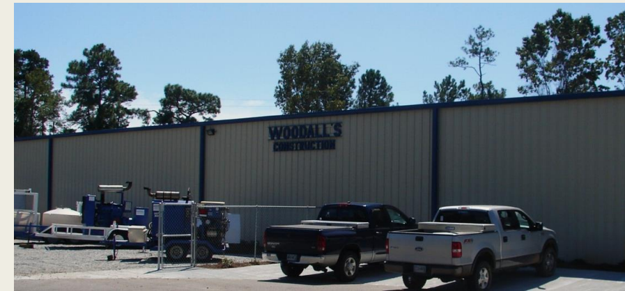
Woodall Const. along Palmetto Commerce Pkwy
